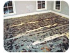
*A proper vapor retarder for solid wood on a slab is always required. In a potentially wet environment, use this system of asphalt mastic and 6-mil poly.*
