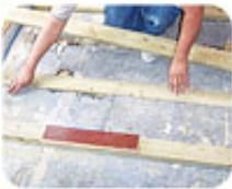
*The contractors are placing solid shims under the sleepers to make the floor flat. This prevented a potential problem.*
