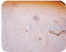
*These high concrete nails were present throughout this room. The flooring was loose and noisy. This floor had to be taken up and new flooring installed after the nails were cut down.*
