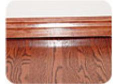
*A nearly 1/2 inch depression along the wall in about 4 feet. The flooring and subflooring would move when walked on.*
