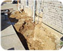
*The trench for mechanicals supplied water under the slab all the way to the powder room. Flooring that had buckled in the hallway was removed.*
