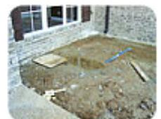
*Note the puddle, the downspout; flooring that had buckled along this wall had been removed.*
